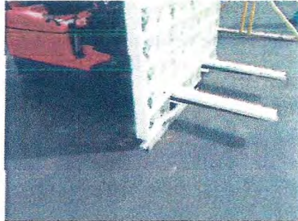
Panel is lifted from shipping crate.
