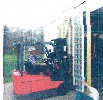
Panel is moved to location.
