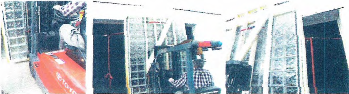
Carefully align panel on all sides before moving into framed opening.
