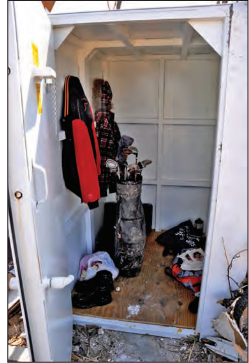
Figure B1-4. Safe room with items stored inside; such items take up space and reduce occupant capacity (Joplin, MO)
