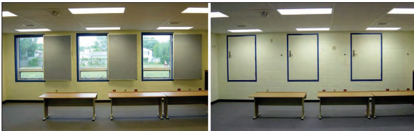
Figure A4-5. Interior operated safe room shutters in multi-purpose classroom/safe room. Image on left is normal usage; image on right shows shutters in 'lock down' position where they are closed and latched
