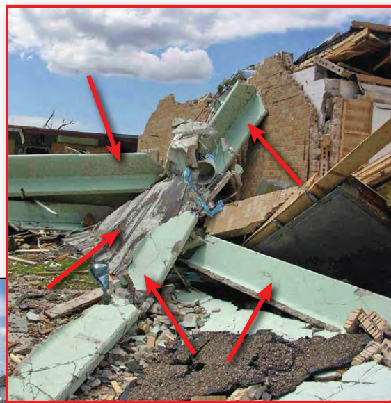
Figure B8-6. Large debris: Roof precast twin tees (red arrows) blew off a hospital and struck another portion of the building (see inset; yellow arrow shows direction of view). One of these flew approximately 80 feet. The building damage at this site was indicative of an EF3 tornado.
