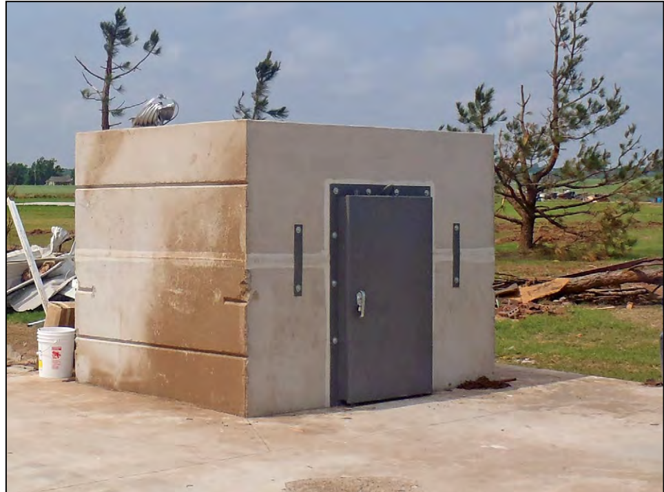
Figure B1-3. Single-use residential safe room after an EF5 tornado (Newcastle, OK)
