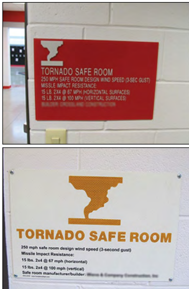
Figure B1-6. Examples of design information signs; though these include Missile Impact Resistance information, such information is not required
