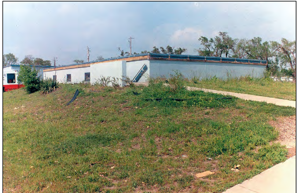
Figure B3-10. View of a community shelter that is partially below grade (Wichita, KS, 1999 tornado) (SOURCE: FEMA P-342)
