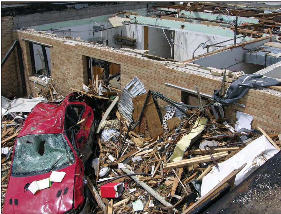
Figure B8-10. Representative quantity, size, and type of debris that is often generated by a strong or violent tornado. The building damage at this site was indicative of an EF3 tornado. (Greensburg, KS, 2007) (SOURCE: FEMA P-577)
