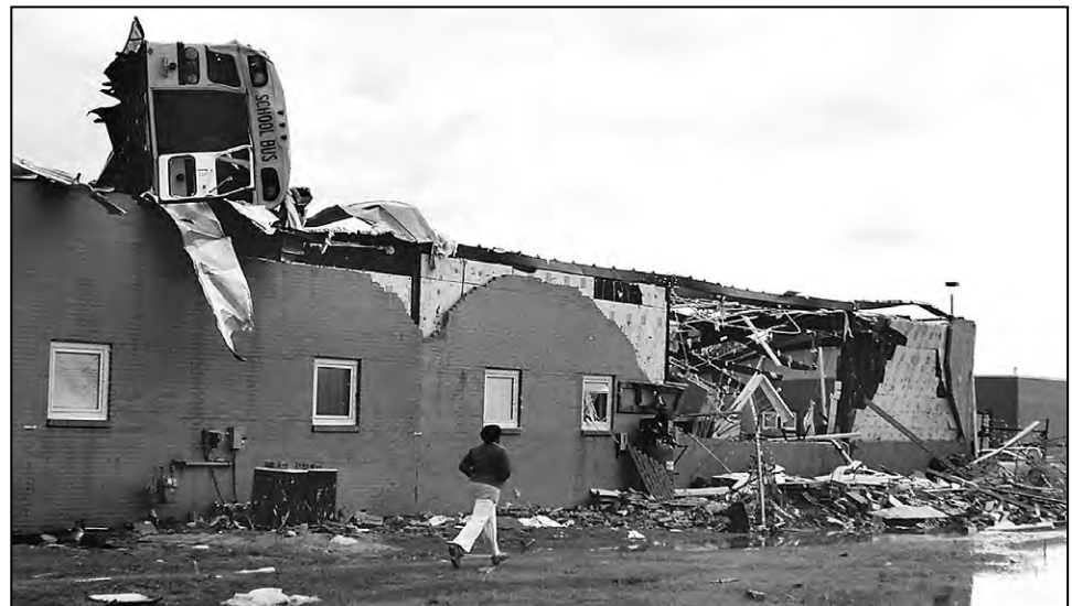
Figure B8-8. Large debris: A school bus was lifted atop a school. (Caledonia, MS, tornado, 2008)
