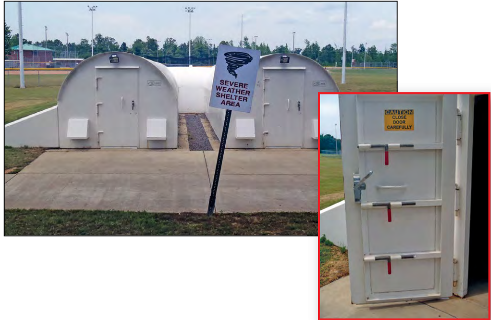
Figure B1-2. Prefabricated steel single-use community safe room (Brookwood, AL)
